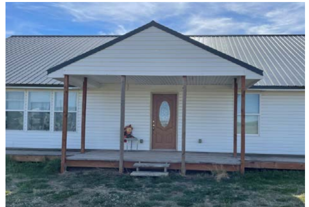
Fort Belknap Teen Safe House (exterior)
